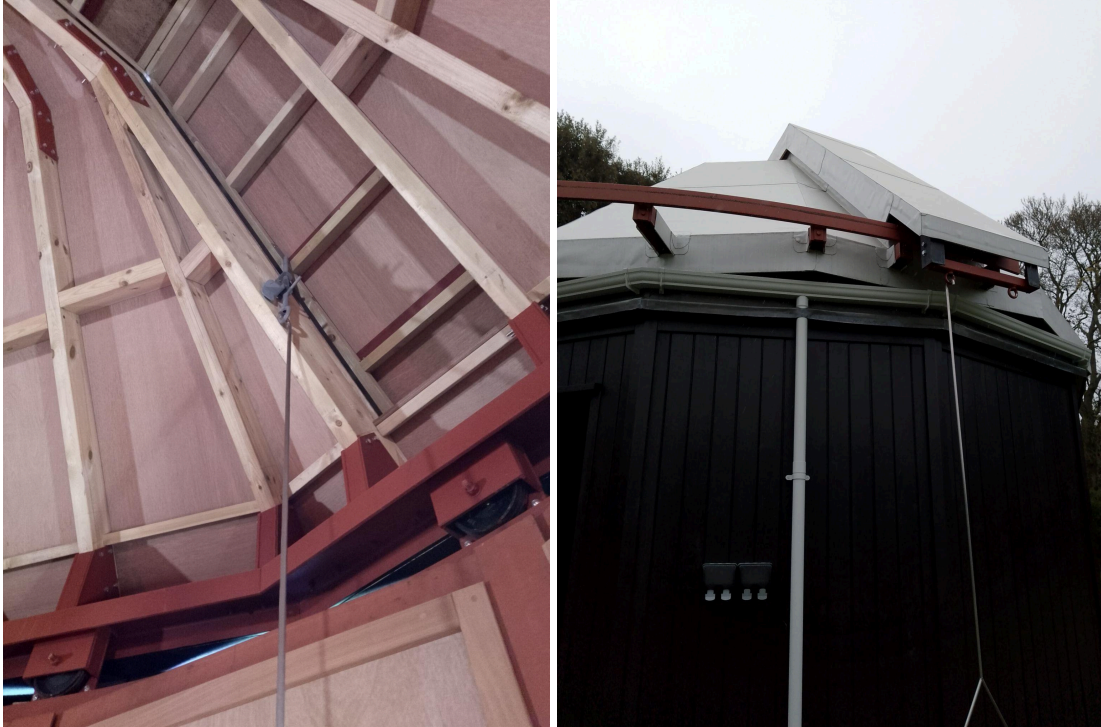
Photos showing how the hooked pole can be used to unlock (left) and move (right) the lid of the slit. The pole is quite heavy and a bit fiddly to fit into the holes, so be careful!
