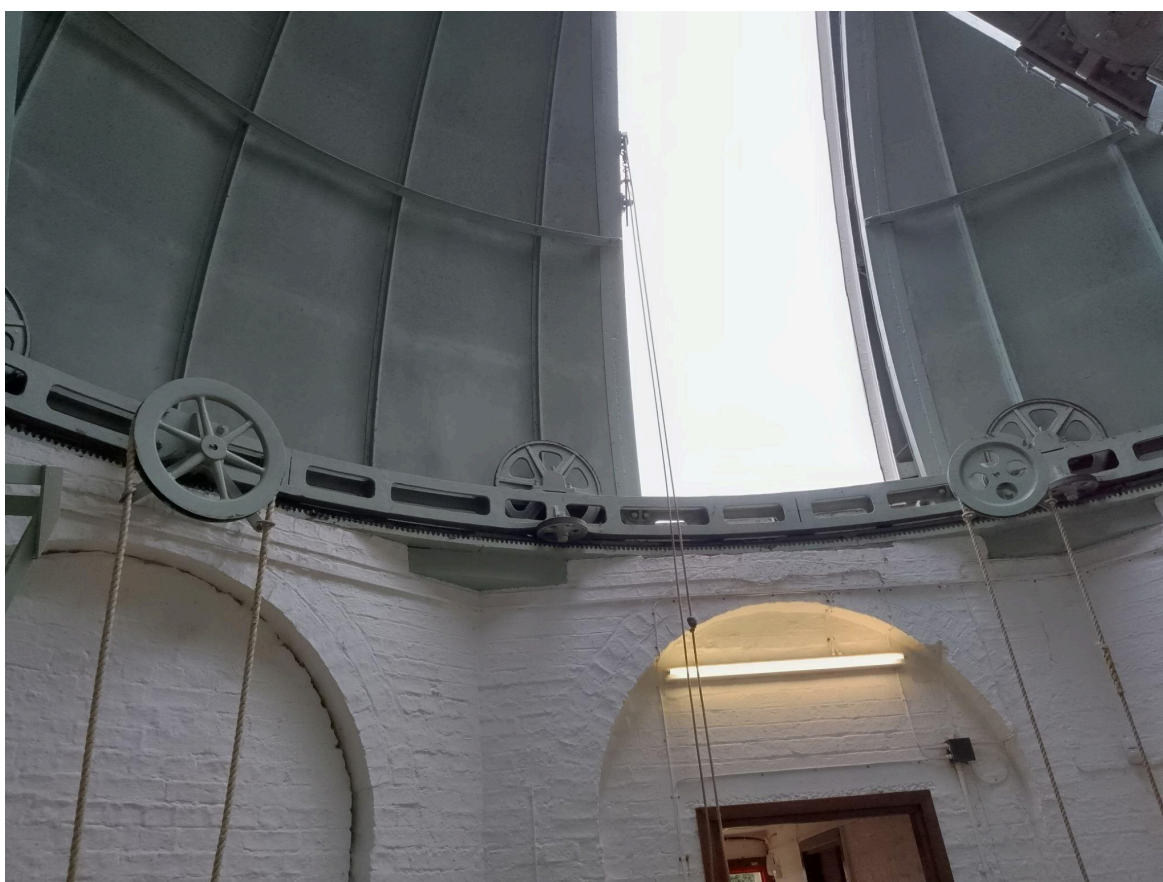
The three ropes for controlling the dome. From left to right: Large rope and pulley for rotating the dome. Small rope and latch for unlocking/locking the slit. Medium rope and pulley for opening the slit.
